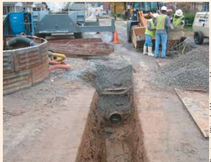
A crew installs 12-inch water pipes in Atlanta, where city officials committed $3.9 billion to overhaul the water and wastewater systems.
